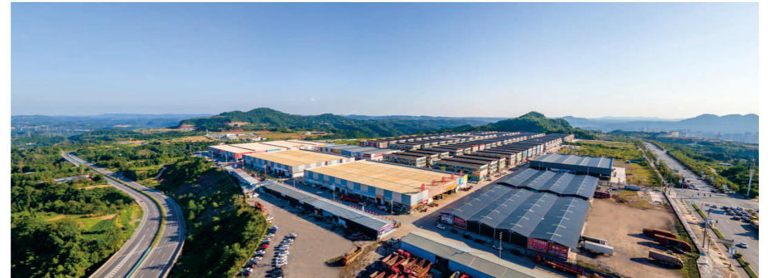
盘兴物流园 Panxing Logistics Park
